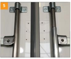
Start by pre-drilling with a 4-mm drill bit. This must be drilled right through if possible.
