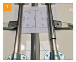
First, it is necessary to check whether the lock to be installed fits in the place where it is to be installed. **Watch out for bars in the door!** Use masking tape to keep the templates in place.
