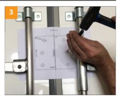
You can now definitively place the template in the required spot. The template has a centre line which must be aligned with the separating line be-tween the 2 doors. NOT on the ends of the rubber.
