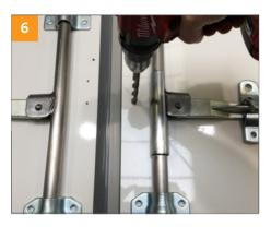
The holes must be drilled out to 11 mm so that the threaded rods pass through the holes. This must be drilled right through too, keeping the drill as straight as possible.
