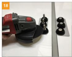
The protruding threaded rod must be ground off first, because red caps will be fitted on it later.
