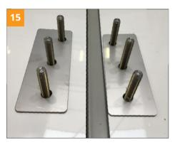
Stainless steel plates are placed over the threaded rods (provided in the kit) on the inside of the door. These plates ensure that pressure is distributed on the door evenly.
